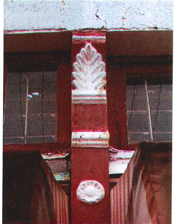
Cast-iron pilasters should be painted to highlight their decorative features such as at 323 Trenton Street.
