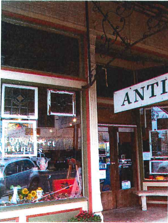
The cast-iron pilaster at 207 Trenton Street are important structural and design elements to the building.
