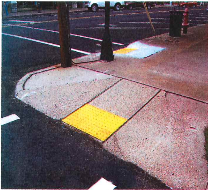
Downtown should be made as ADA compliant as possible. These types of curb cuts should be added along Commerce, Cotton and Wood Streets as well as along Trenton Street.
