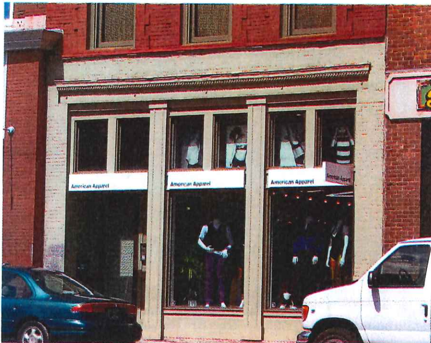
New display windows should be appropriately designed and with clear glass such as shown above.
