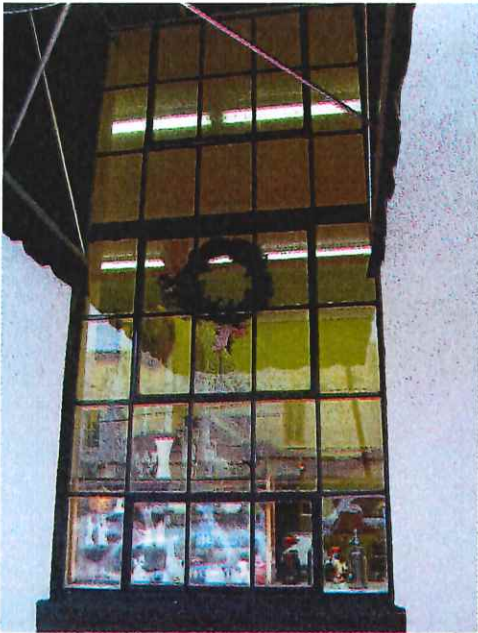
This historic metal window should be repaired as needed and retained (301 Trenton Street).
