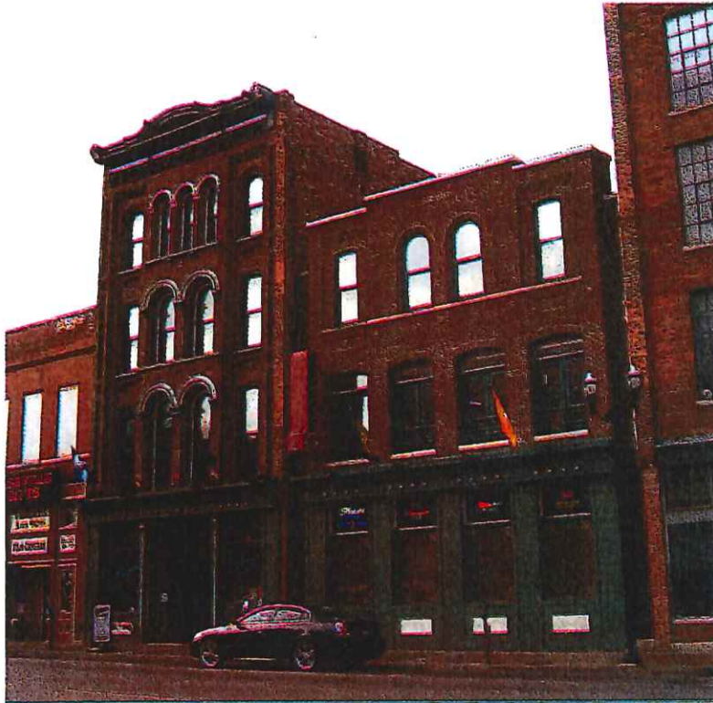
The new building pictured on the right appropriately used materials similar to those of its neighbors in its maroon brick construction, wooden window sashes, clear glass window panes, and wooden storefront.
